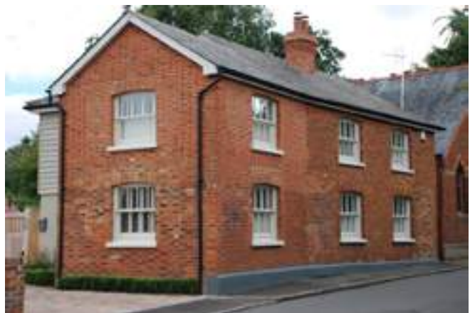
Extension and conversion – The Street
