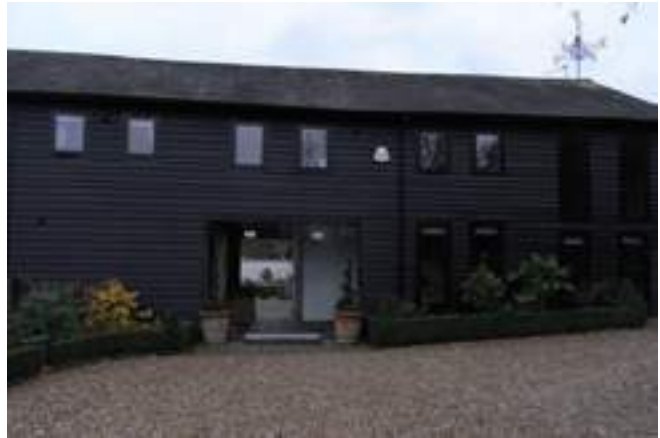
Barn conversion – Gravelly Lane
